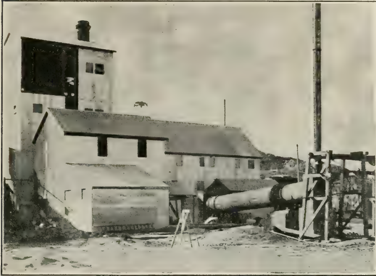
FIG. 76.—DRYING FURNACE, PLANT NO. 2, SULPHIDE CORPORATION.
